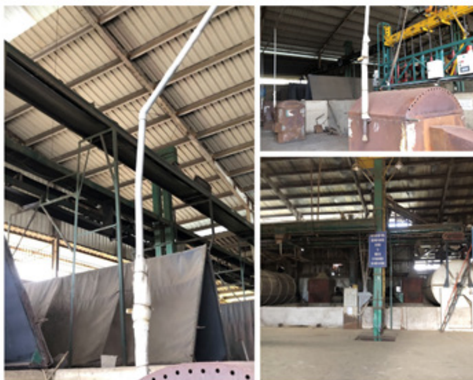
Photo 15. Using biogas from wastewater treatment for drying coffee
