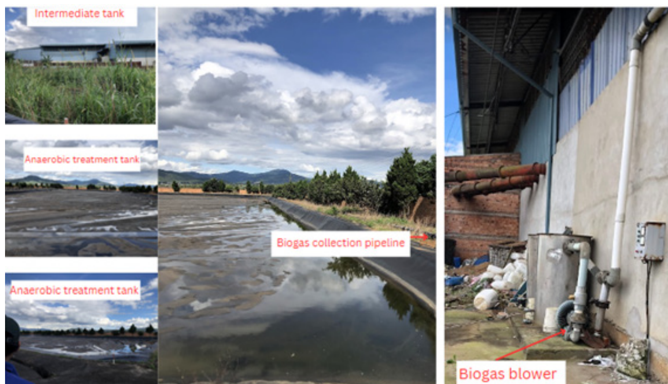
Photo 14. Converting wastewater into biofuel for coffee drying or electricity generation
